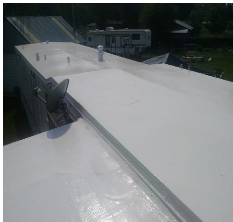
2015 Veteran Roof Coating Non Profit Project
